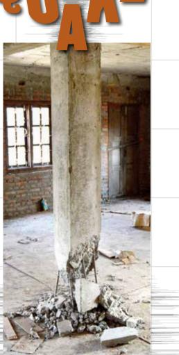
The Purdue team documented damage such as this case of combined shear and axial (compressive) failure of a column.
